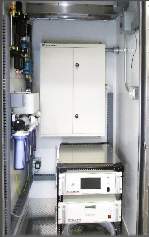
Interior 3300Xi HgCEMS Cabinet
